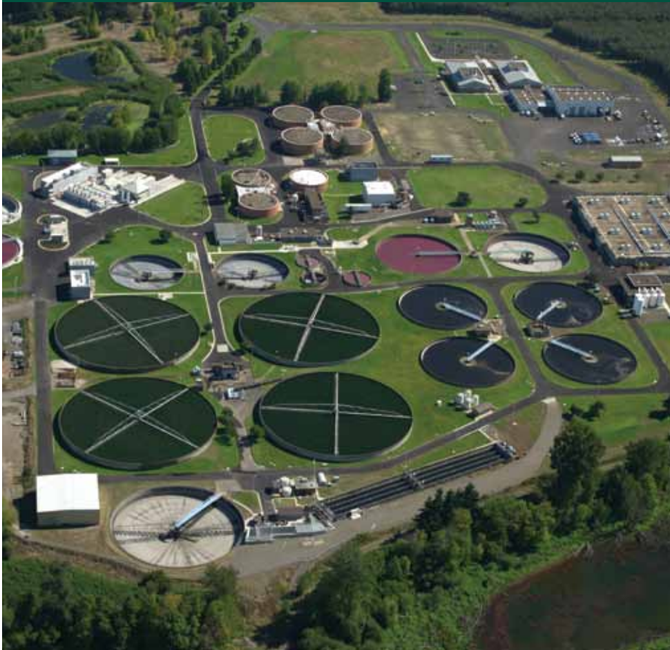
Salem's wastewater treatment facility
