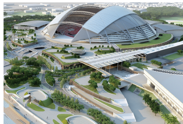
An artist's depiction of the Singapore Sports Hub now under construction.
